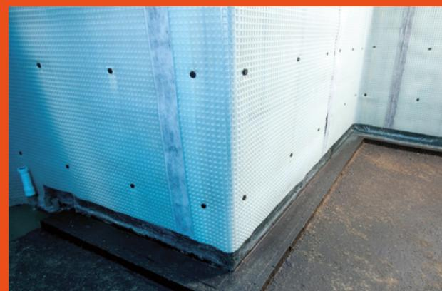
Engineering brick detail housing perimeter drainage, with non-return odour resistant valve awaiting fitting (far left)
