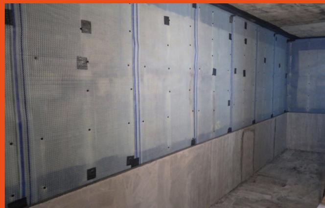
Swimming pool recessed into lower basement level floor. Perimeter drainage channel at floor level runs around top of pool liner wall. Pool walls and floors are waterproofed with an elastomeric cementitious slurry system and fillet sealing detail at wall/floor joints.
