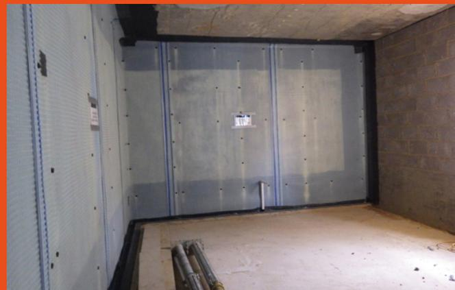
*Upper basement level showing 8mm cavity drain membrane to walls and banded perimeter drainage channel.*
