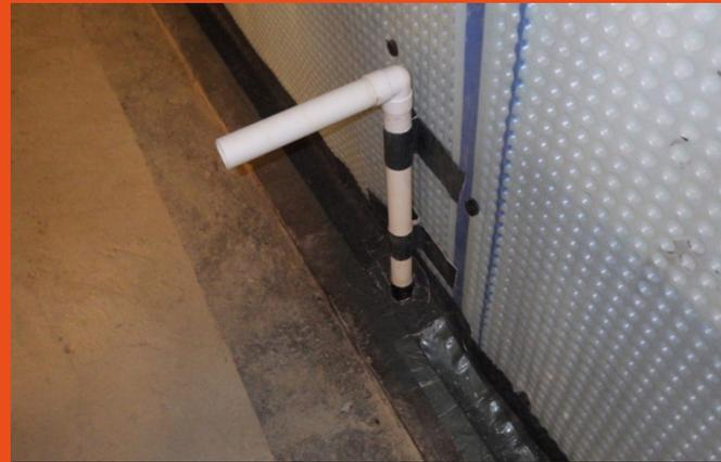
*8mm cavity drain membrane to wall at upper basement level with perimeter drainage channel sealed with liquid applied waterproofer and corner strip, showing access point via 40mm pipe and 90° bend.*
