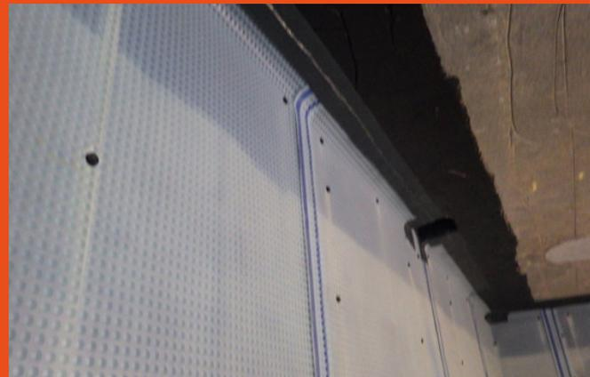
*Lower basement level showing 8mm cavity drain membrane on wall to soffit detail sealed with liquid applied waterproofer. 40mm discharge outlets drain down from the level above and angle back towards perimeter liner wall.*
