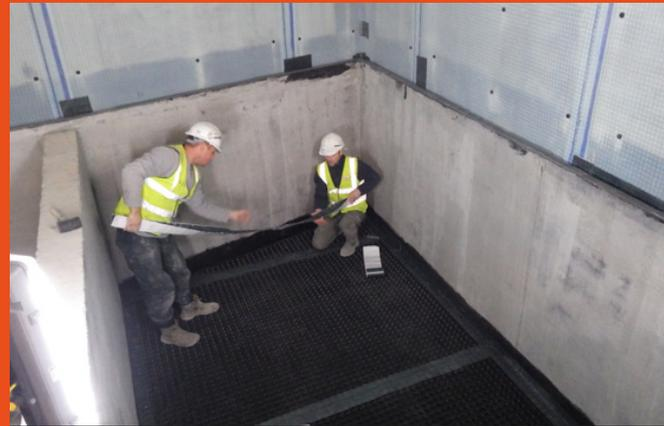
Service trench waterproofed with a cementitious slurry system and 20mm cavity drain membrane to floor. Lower basement level drainage channel runs around upstand of trench liner wall and discharges behind wall down to perimeter drainage channel set in trench floor slab.
