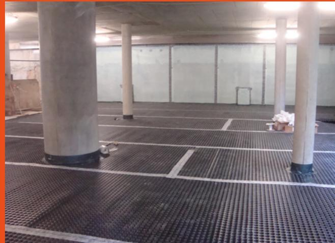
*The Grade 3 section of the basement, waterproofed with cavity drain membranes, will be used as a retail space*
