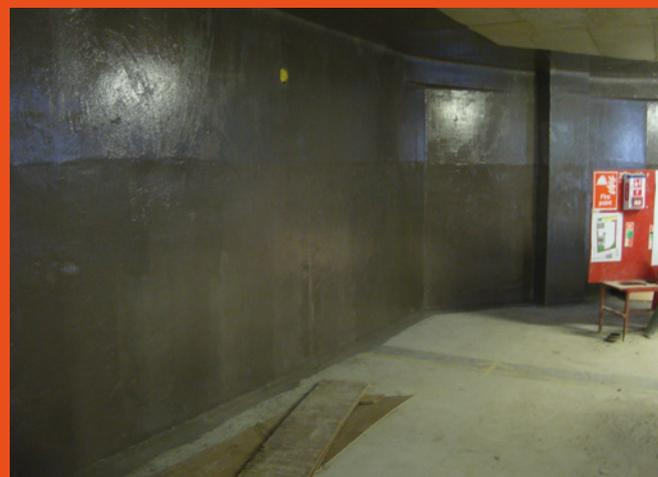
*Walls in the plant room section were waterproofed with liquid epoxy waterproofer*
