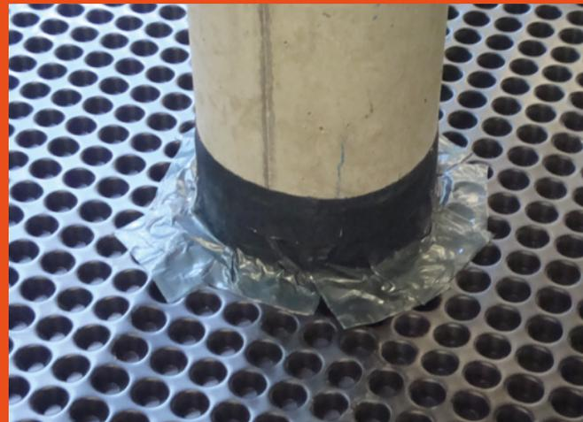
*Sealing detail using liquid epoxy waterproofer and corner strip*
